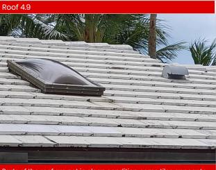
Parts of the roof are not in clean condition, some tiles appear to have been replaced.
