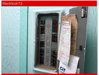
Electrical panel is Federal Pacific, it was last inspected in the year 2012. The panel is in a wooden frame with a picture hanging over if
